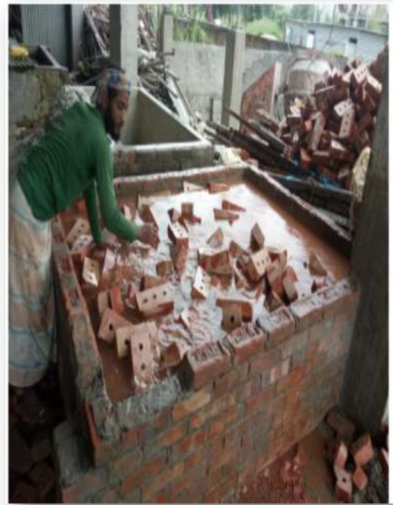
Bricks are Soaking Water
