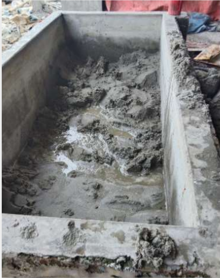
Sand Washing in Water Reservoir
