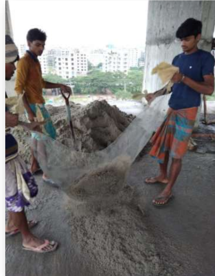
Sand and Cement Mixture Screening by Net
